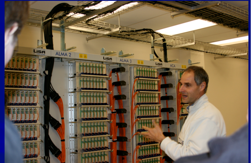
•Fiber Optic patch panel in AOS TB
