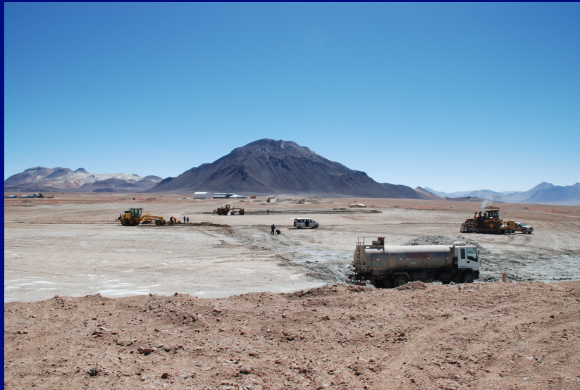
Array Operations Site Technical Building
