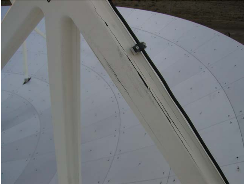
Figure 2. Section of damaged feed leg.
