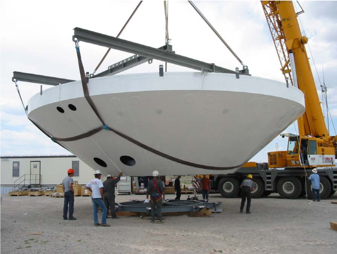
Figure 5. Lifting assembled BUS onto the mounting fixture.
