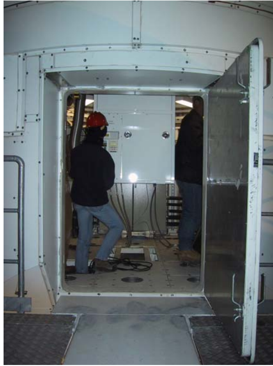
Figure 12a. Evaluation receiver #1 installed in antenna cabin
