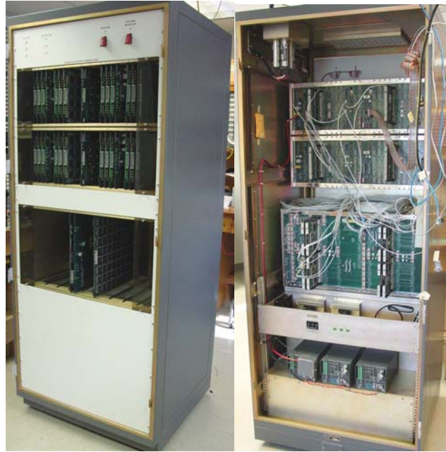
Figure 20. Front (left) and rear of prototype 2-antenna correlator rack showing card cages, cards, backplanes, fans, and power supplies mounted.
