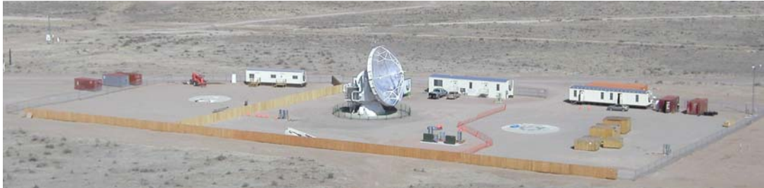
Figure 6: Completed antenna foundations at ATF site as of March 12, 2003.
