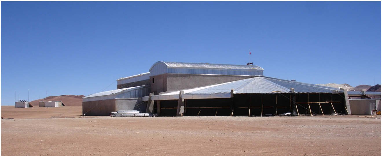
The Array Operations Site (AOS) Technical Building, which will house array elements such as the ALMA Correlator. © NAOJ
