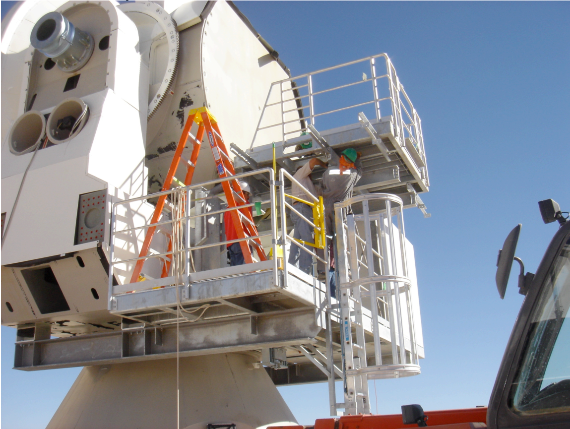
Figure 2 The access platforms were being installed on the VertexRSI antenna at press time.
