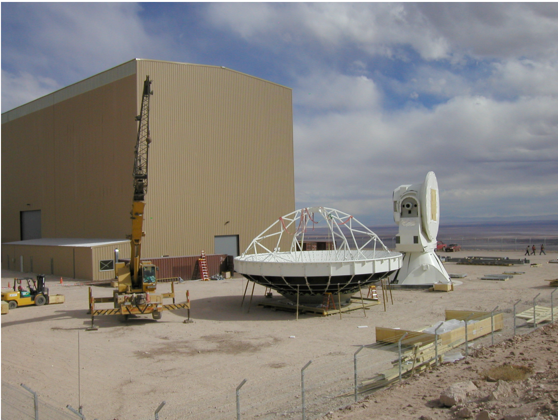
Figure 1 The first ALMA production antenna reached the OSF and assembly was begun. Here the VertexRSI pedestal stands on its pad to the right of the partially assembled backup structure in front of the site erection facility at the OSF.
