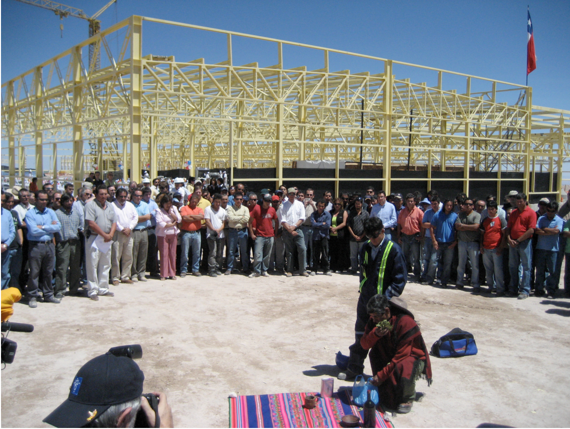
Figure 3 During the celebration of the completion of a roof on the OSF warehouse, members of the local community joined ALMA and others as a pachamama or 'payment to the Earth' ceremony was held, in which harmony is sought. Photo: R. Simon
