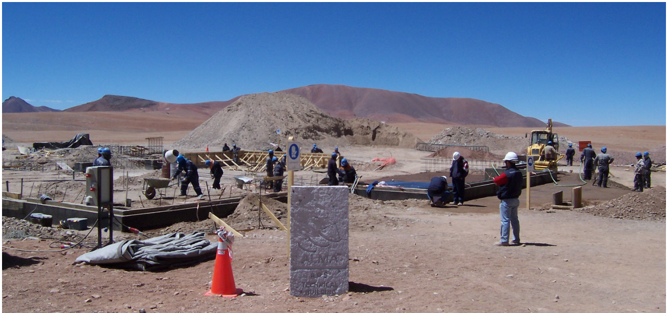
Construction in progress on the correlator building (5000m), December 20, 2005.
