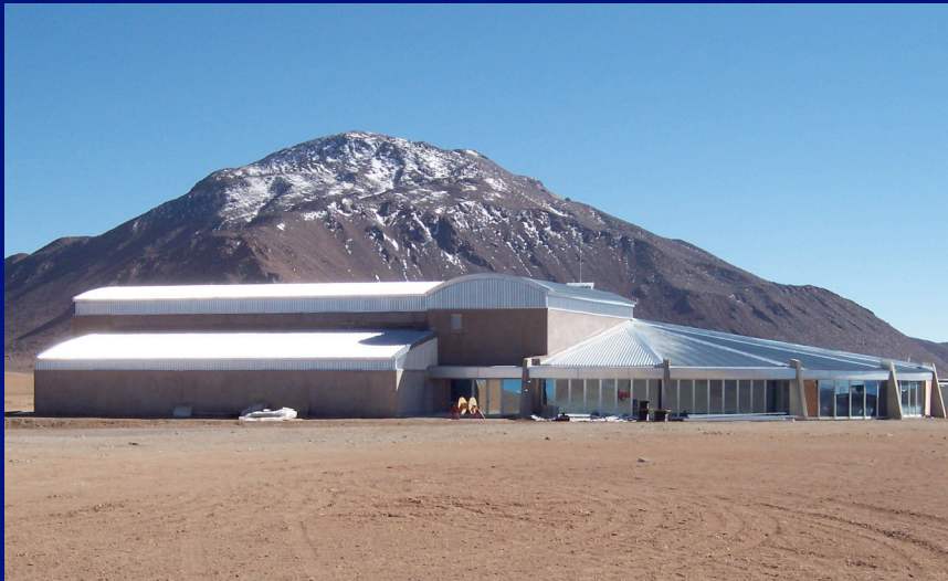
Array Operations Site Technical Building
