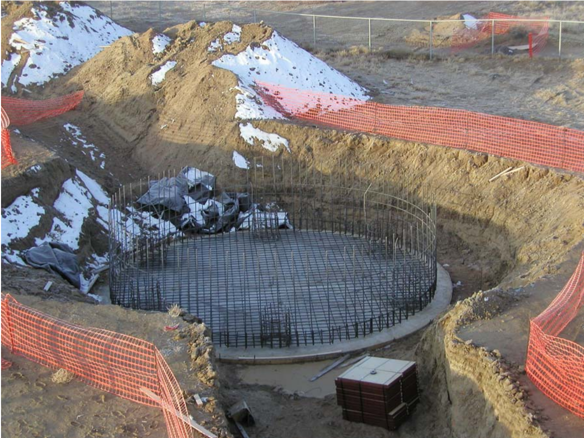
Figure 10. The NAOJ foundation as of December 6, 2002.
