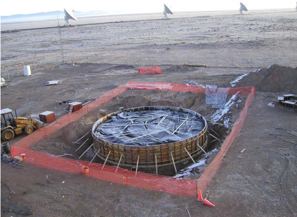
Figure 9. The AEC foundation as of December 6, 2002.
