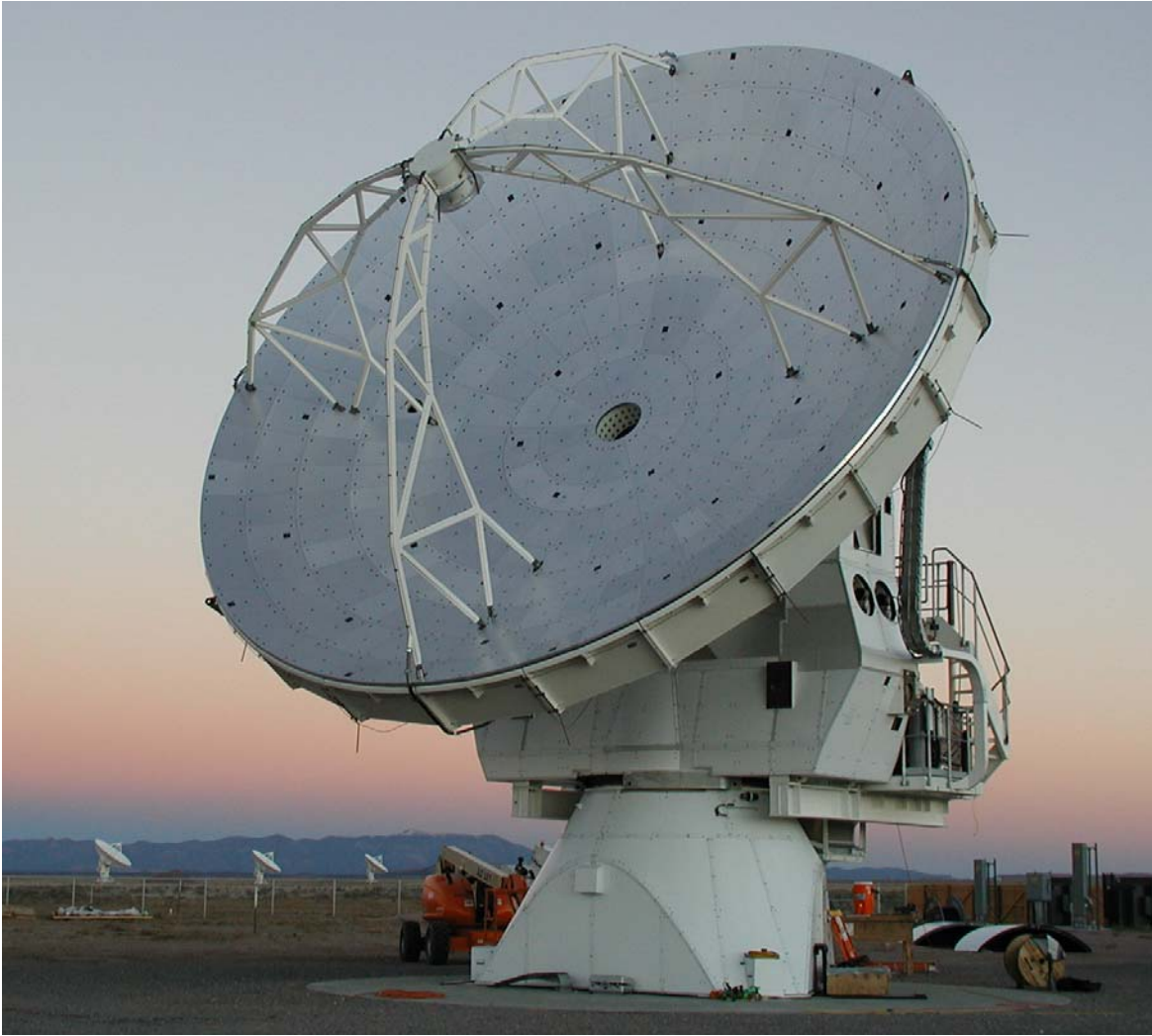
Figure 7. The VertexRSI antenna – assembled with panels installed.
