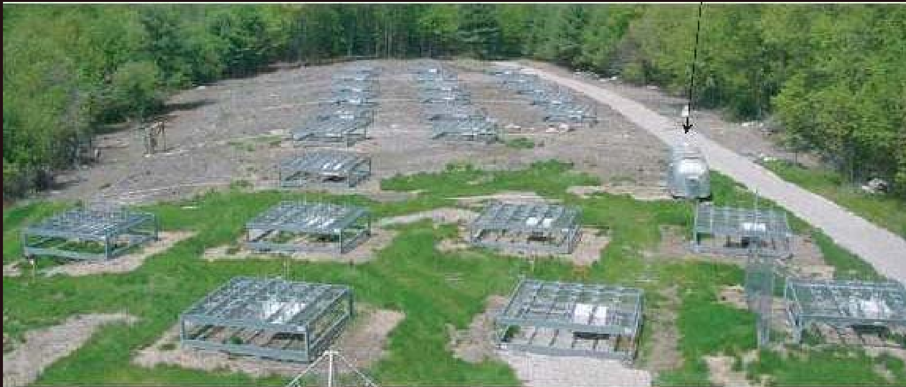
Overall view of the 25 5x5 crossed dipole stations of the Deuterium array
