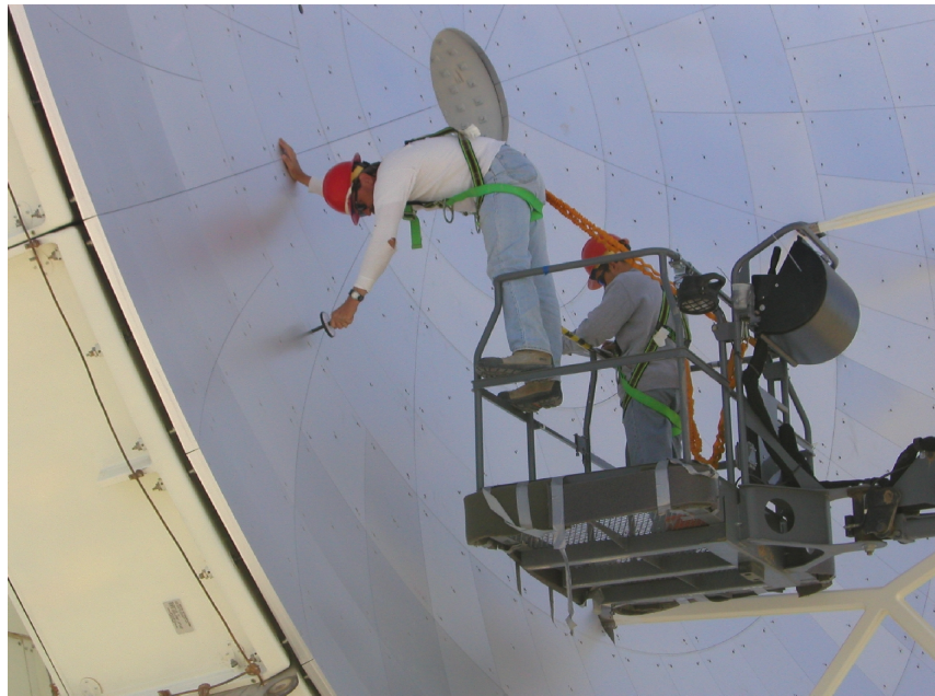
Figure 14: Panel adjustment of the VertexRSI prototype antenna.
