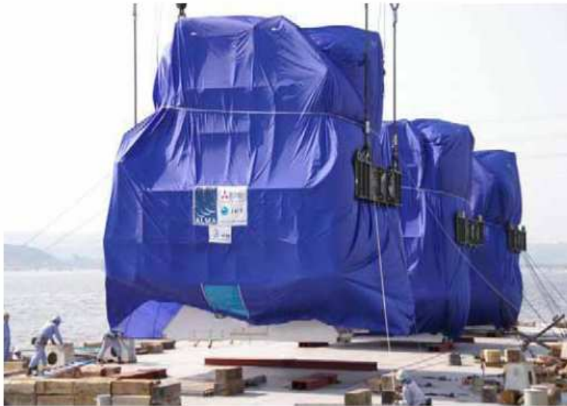
Loading to Barge
